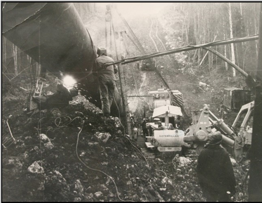
Soviet Pipeline Construction. Source: Gozprom.com
